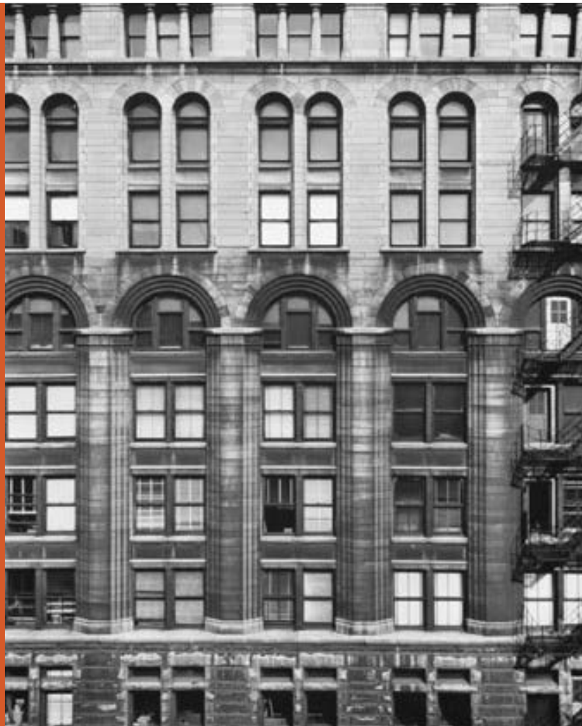
Richard Nickel, Auditorium Building , Chicago, Illinois, c. 1955
